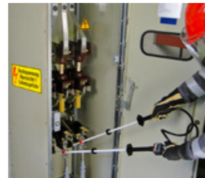
Test with HS 11 at 10 kV transformer
